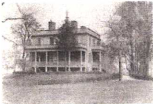
HISTORIC PHOTOS - HAMILTON GRANGE ON ORIGINAL SITE
